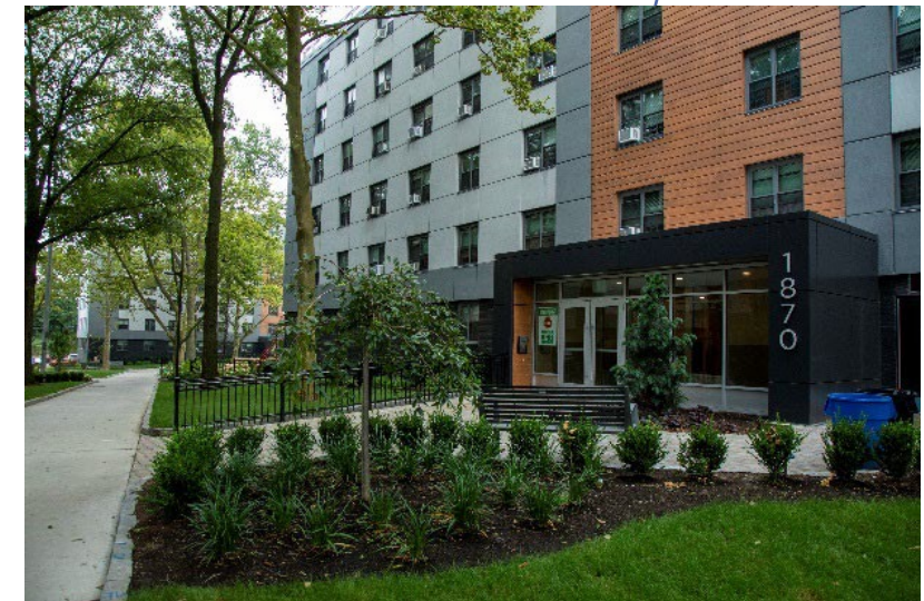
Site improvements at Baychester
