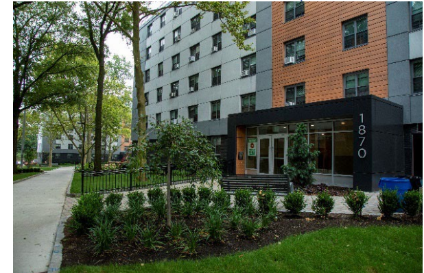
Site improvements at Baychester
