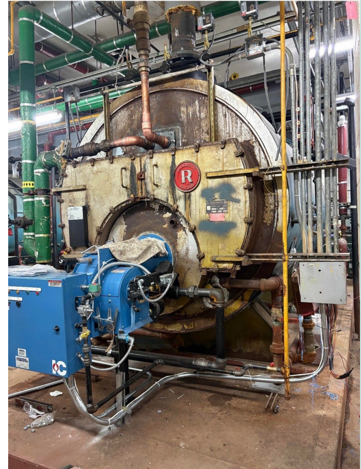
SGL boiler after renovations.
