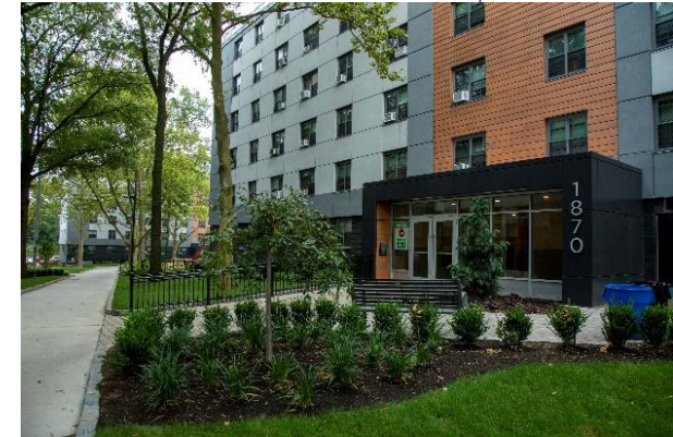
Site improvements at Baychester
