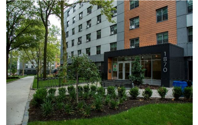
Site improvements at Baychester
