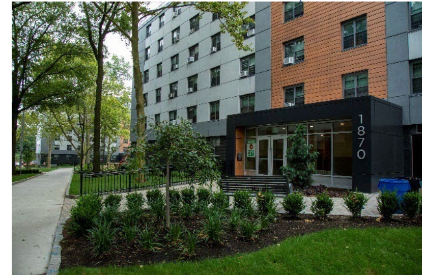
Site improvements at Baychester
