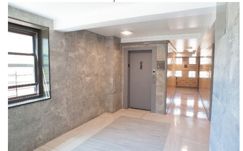
Renovated building entrance at Ocean Bay (Bayside)
