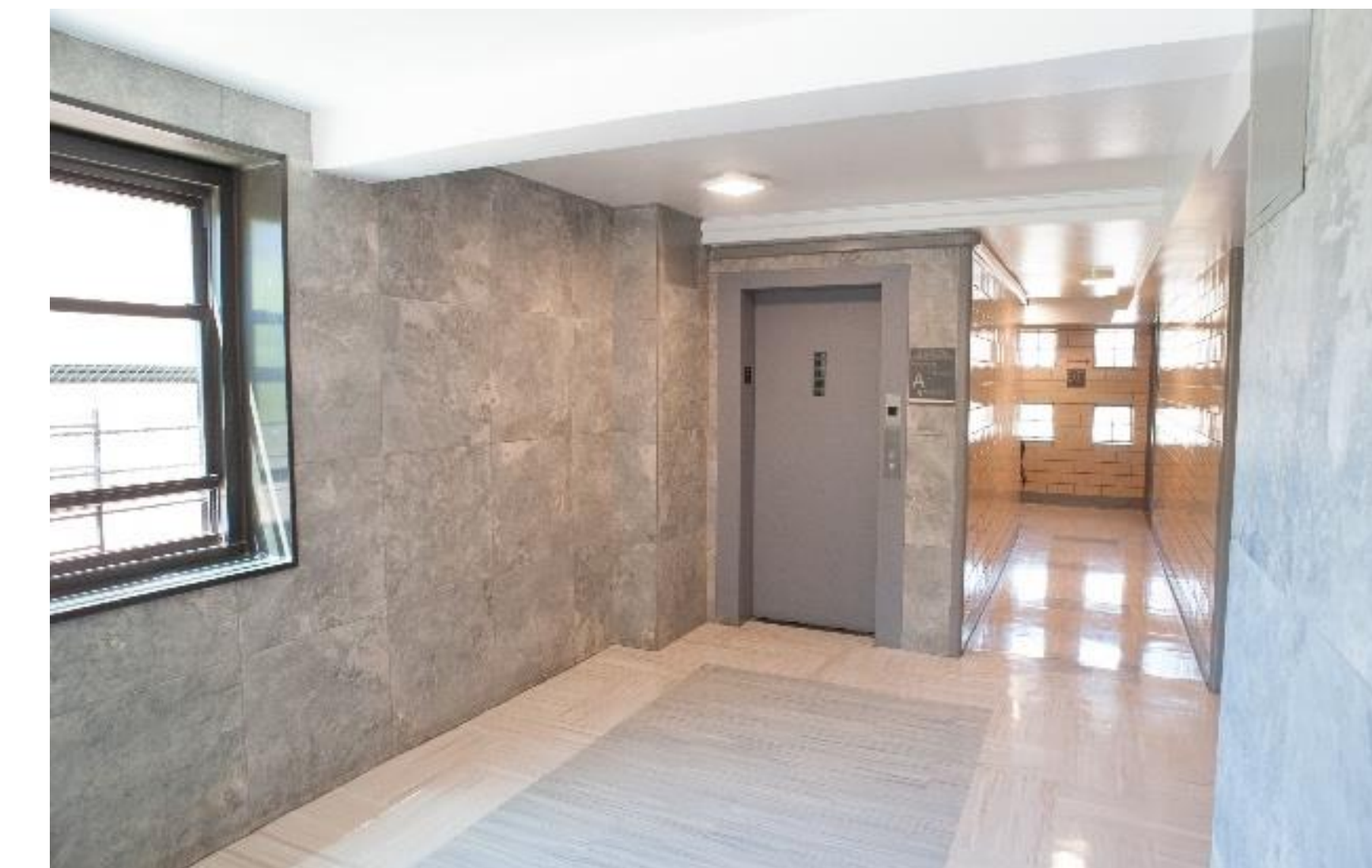
Renovated building entrance at Ocean Bay (Bayside)
