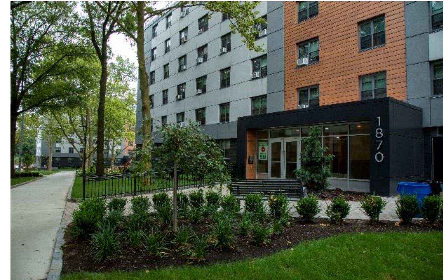
Site improvements at Baychester
