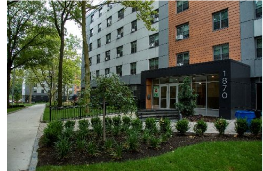
Site improvements at Baychester
