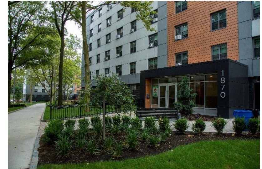
Site improvements at Baychester
