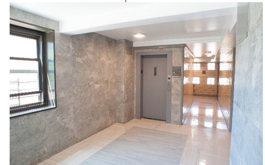
Renovated building entrance at Ocean Bay (Bayside)
