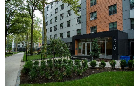
Site improvements at Baychester
