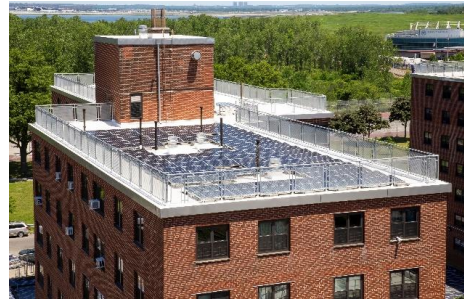
Repaired roof and solar panel system at Ocean Bay (Bayside)
