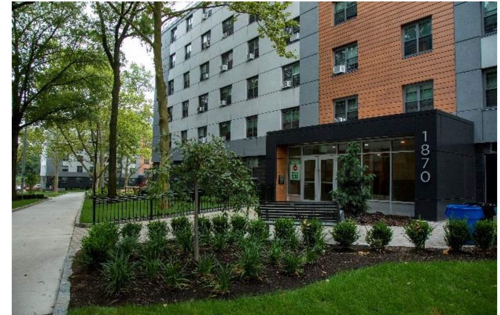
Site improvements at Baychester
